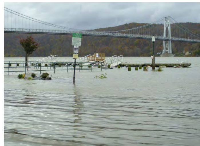
FIGURE 6. POUGHKEEPSIE WATERFRONT FLOODING AFTER SUPERSTORM SANDY IN 2012. PHOTO SOURCE: DCTC.
