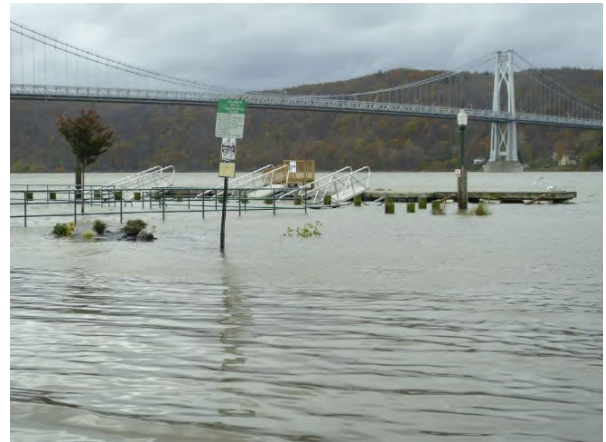
Figure 1. Poughkeepsie Waterfront flooding after Superstorm Sandy in 2012 (Source: DCTC)
