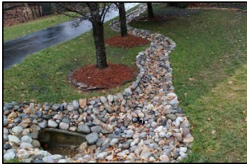
Source: Drainage and Erosion
