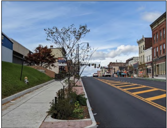
Figure 29. Rain Garden alongside Broadway in Kingston, NY (Source: Duchess County )
