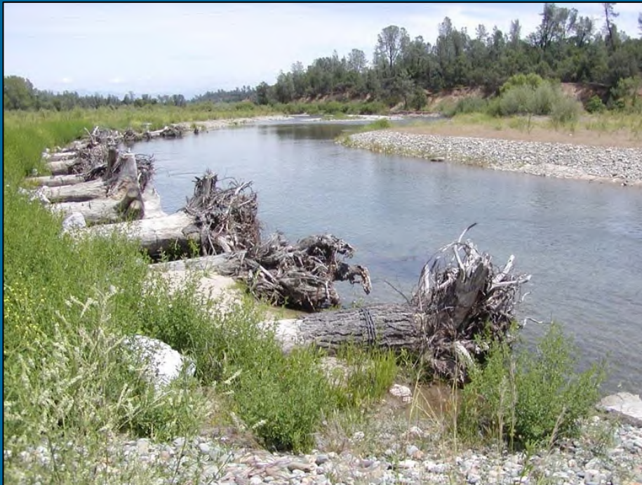
Figure 28. Rootwad revetment in Clear Creek, Redding, CA (Source: VDOT )
