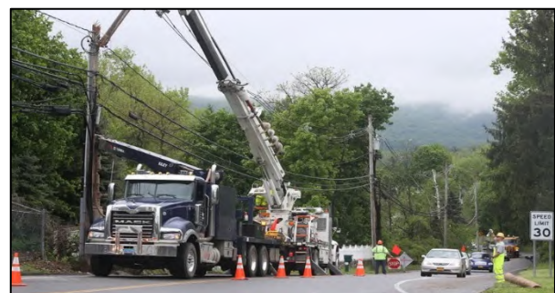
Figure 16. Central Hudson replacing a damaged utility pole following a severe storm (Source: Poughkeepsie Journal )
