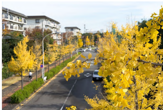
Figure 39. Trees planted between the sidewalk and curb (Source: Treehugger )
