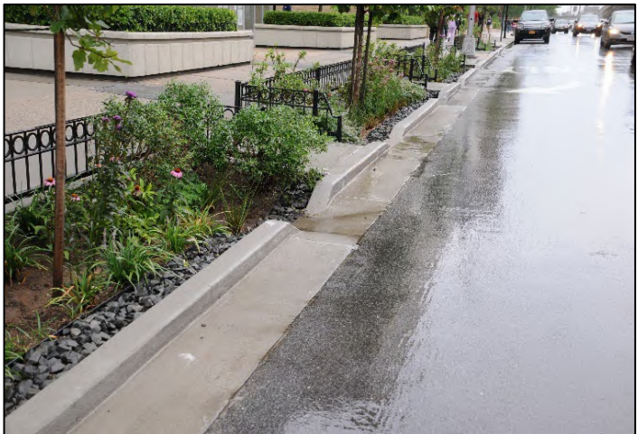
Figure 30. Rain garden alongside a road in Queens, NY (Source: NYC Water )
