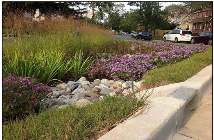
Figure 32. Bioretention example alongside a road in Maryland (Source: Montgomery County of Department of Environmental Protection )
