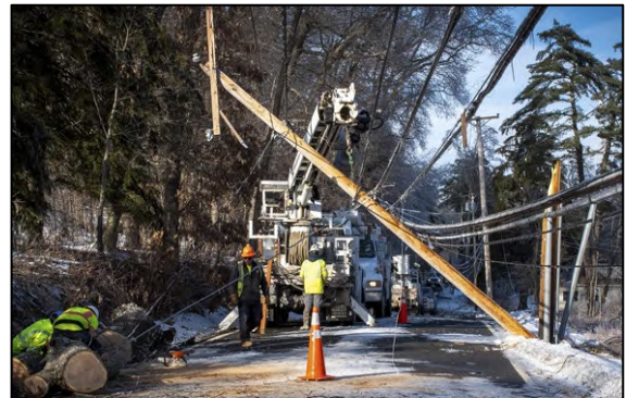
Figure 14. Central Hudson repairing a damaged utility pole blocking the road following a winter storm (Source: Central Hudson)
